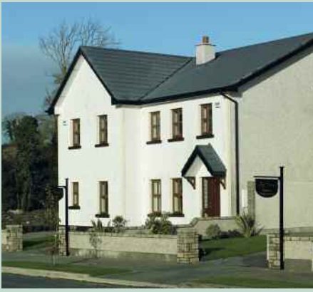
Semi Detached homes , Westmeath (110 m 2 ) Internally Insulated Single Leaf Cavity Block Wall. Similar to Wall 3 .
