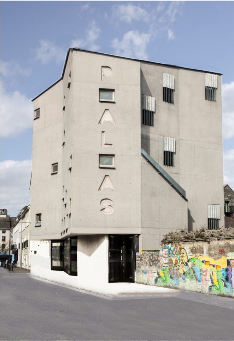
Architectural Concrete, Pálás Cinema Galway
