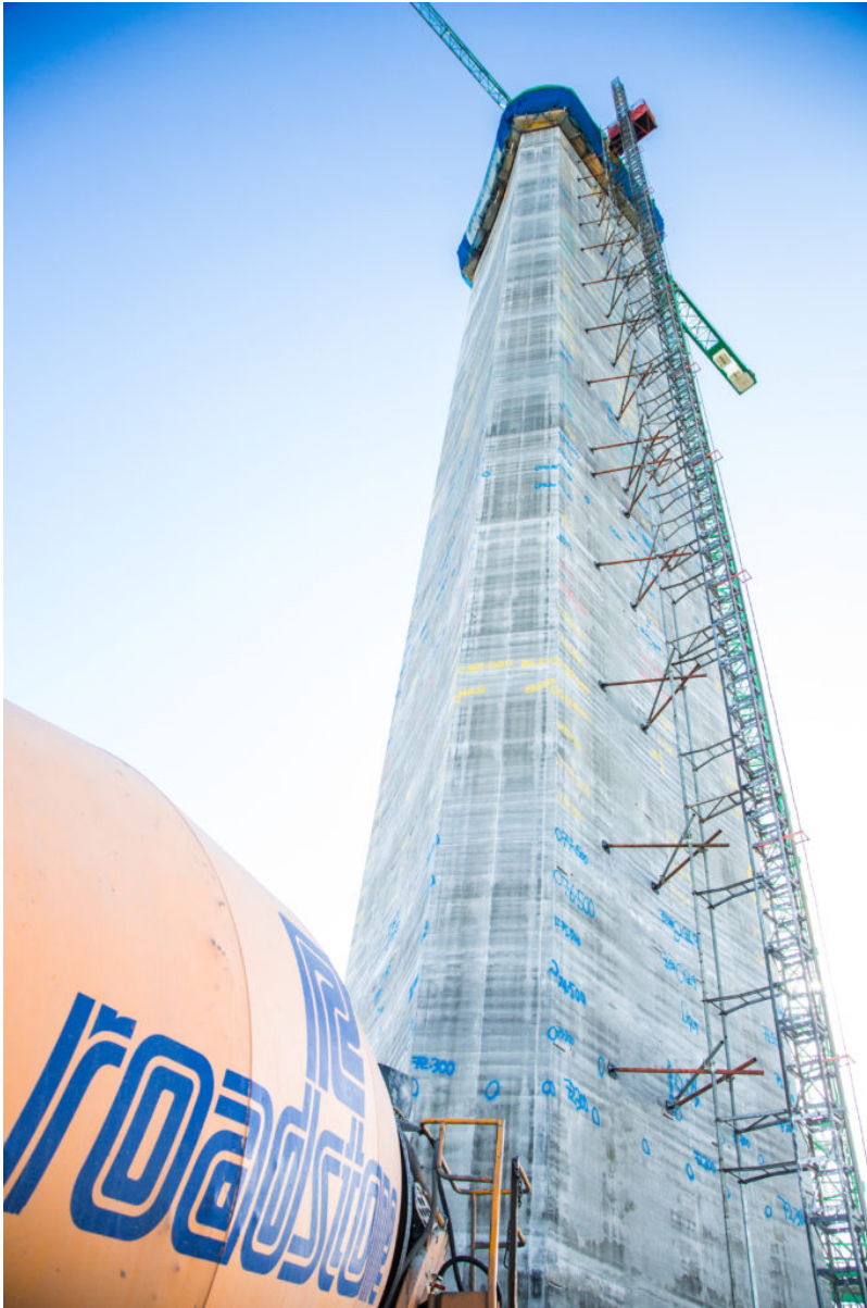
Slipform Concrete, Visual Control Tower, Dublin Airport
